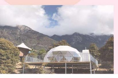
Frame Material: Galvanized steel with hard shell white paint eliminate with strong bases. Outer shell is PVC white non-transparent . PVC door is standard . Unit shown with optional glass door .
